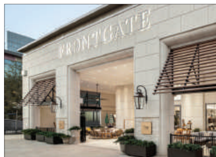
Project: Frontgate Architect: FRCH NELSON Photograph: Richard Cadan / @cadanphoto
